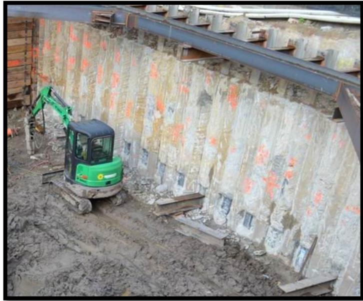
Figure 4.1 – Secant Wall | Courtesy of DAVIS
