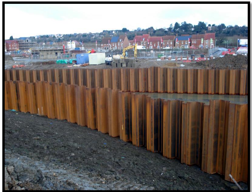
Figure 2.1 – Sheet Piling | Courtesy of Maxx Piling
