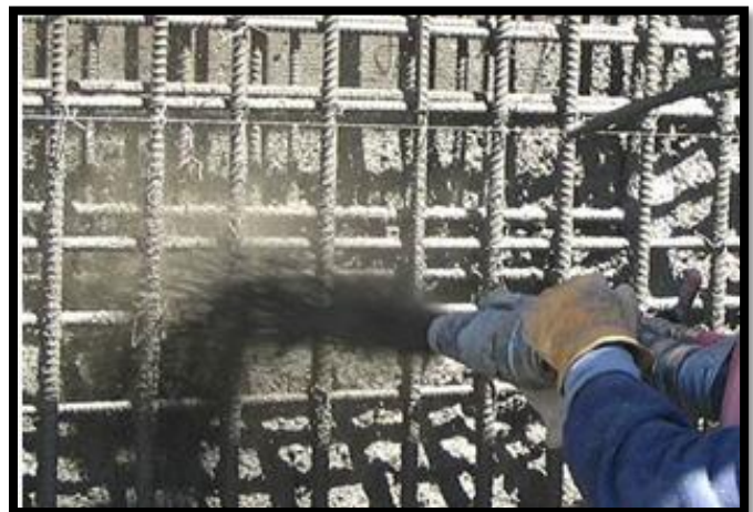
Figure 3.3 – Shotcrete Installation |
